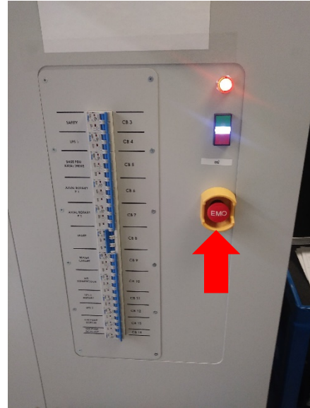
Emergency Power Off Button at the Power Distribution Unit
